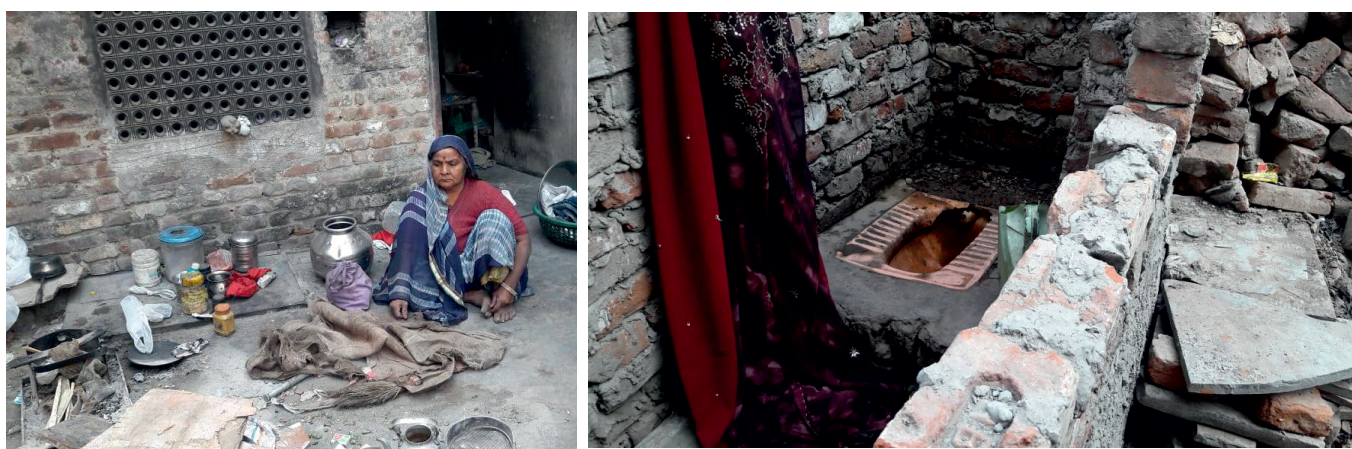
Teeja's Household and the condition of IHHL in her house, Swami Basti.
