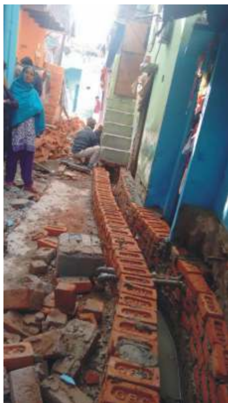
Communities are demanding that drains be constructed in their clusters
