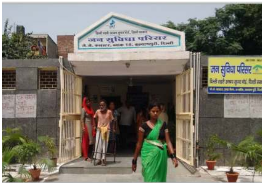
Community Toilet Complex in Trilokpuri Cluster, Delhi
