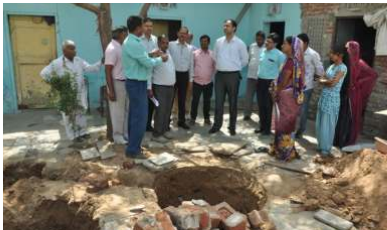
Community representatives were taken to Delhi and Bikaner to observe how two-pit and other types of toilets were constructed
