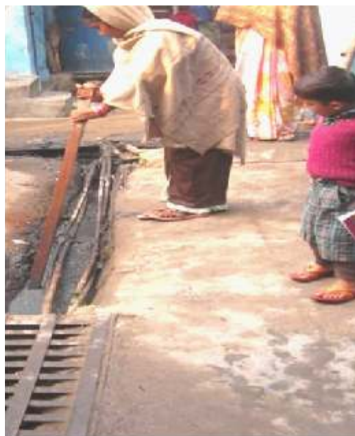
In some clusters people started cleaning the drains themselves
