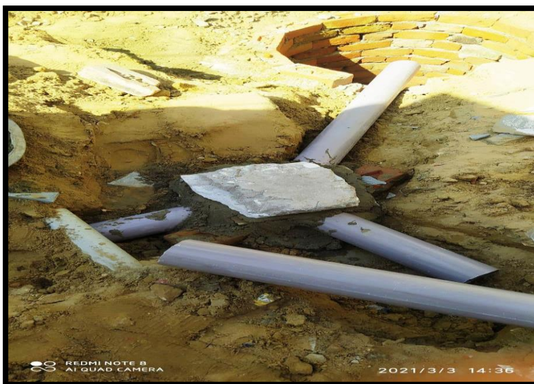
Twin pits construction in Sunder Nagar
