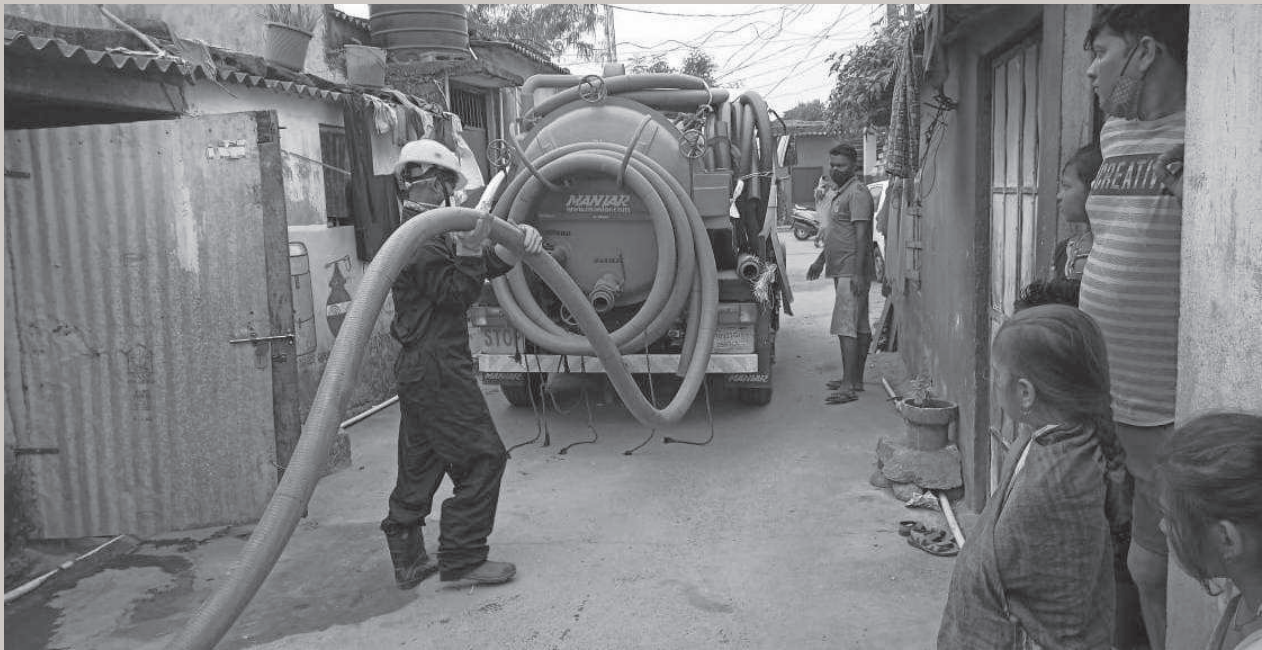
Desludging in progress
